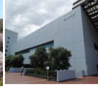
Cafeteria Building (all four floors)
